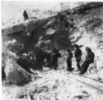
← LEFT: A working face at the Aucanquilcha sulphur mine high in the Chilean Andes. The maximum depth of this face is 66 feet.
